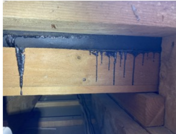
In the Bitumen below metal roofs used as a weatherproofing
