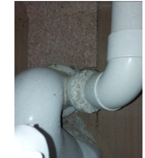
Putty to waste pipe Putty around pipe joint
