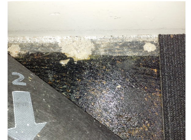
Bitumen based adhesive under flooring
