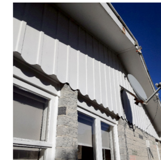
AC soffit and gable Common to many houses
