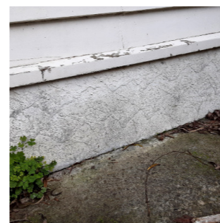
Backing boards Common to many houses particularly state houses
