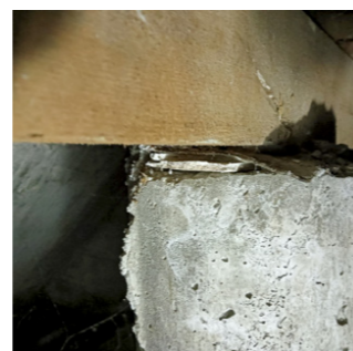
Packing AIB and bitumen Common to houses on piles
