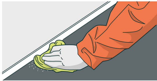
FIGURE 1: Wipe up dust and debris with a damp rag/wet wipe
