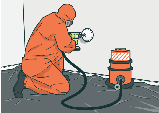
FIGURE 4: Drilling holes in AIB using drill shroud and H-class vacuum cleaner
