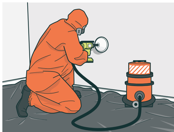
FIGURE 10: Example of using a dust shroud and low speed drill connected to an H-Class vacuum cleaner
