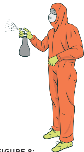
FIGURE 8: Gently wetting ACM before working on it will reduce the amount of dust produced
