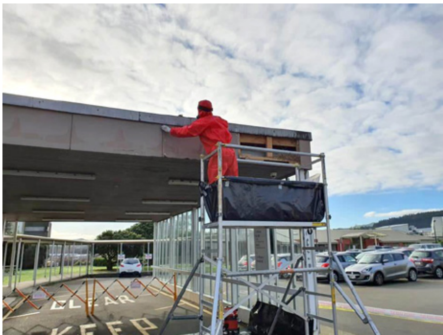
FIGURE 3: Removal work without an enclosure
