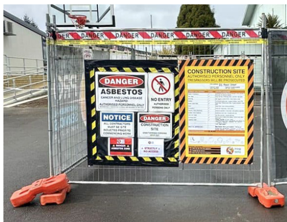
FIGURE 1: Example of solid barrier fence
