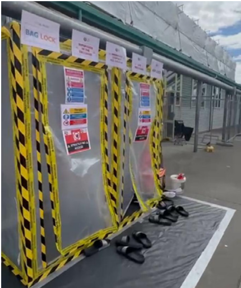
FIGURE 13: Example of airlock and baglock
