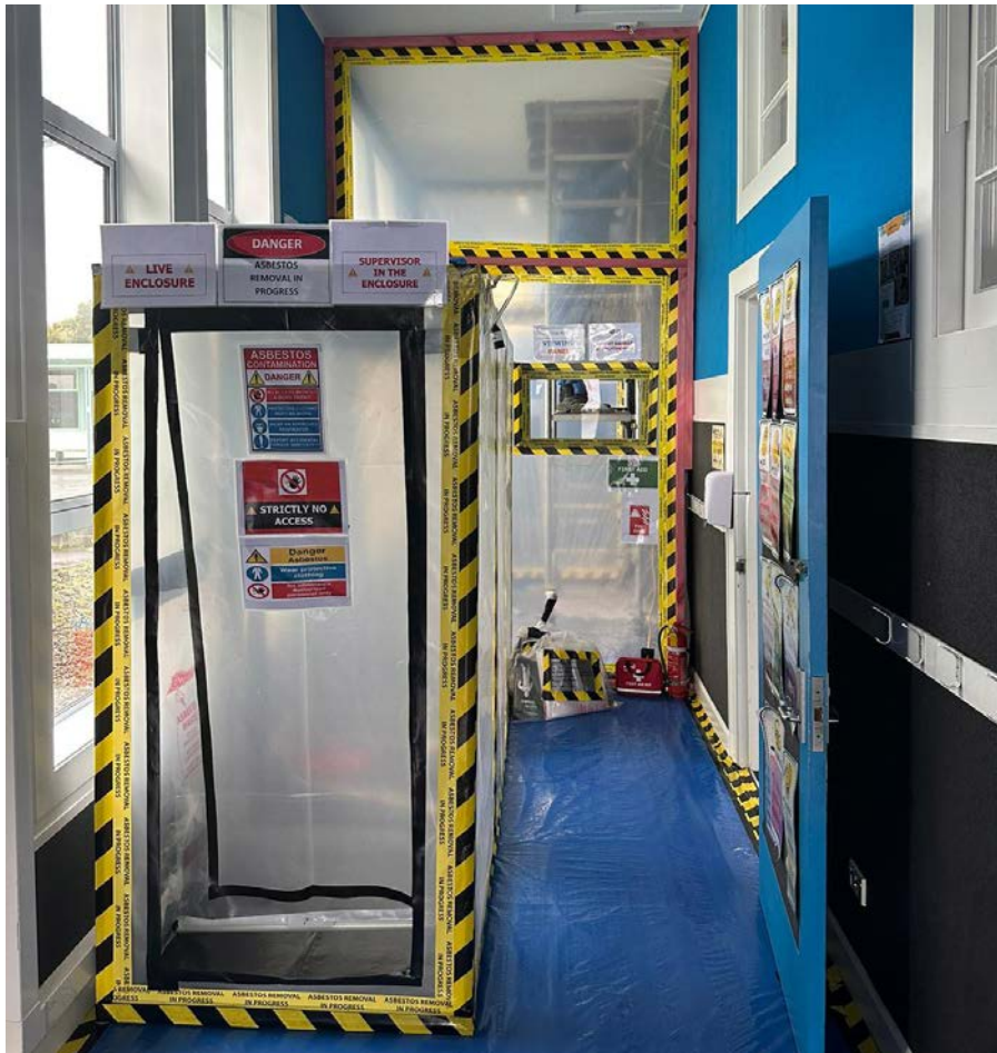
FIGURE 8: Example of an airlock used in transiting
