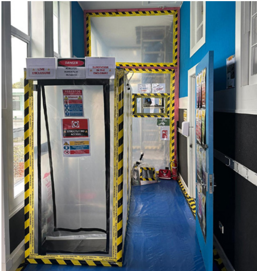
FIGURE 8: Example of an airlock used in transiting
