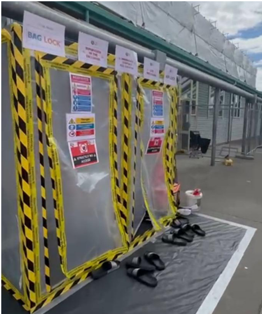
FIGURE 13: Example of airlock and baglock
