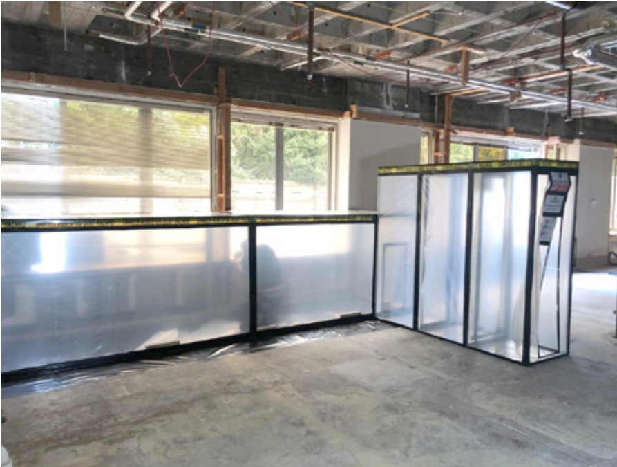
FIGURE 2: Enclosure with three-stage airlock
