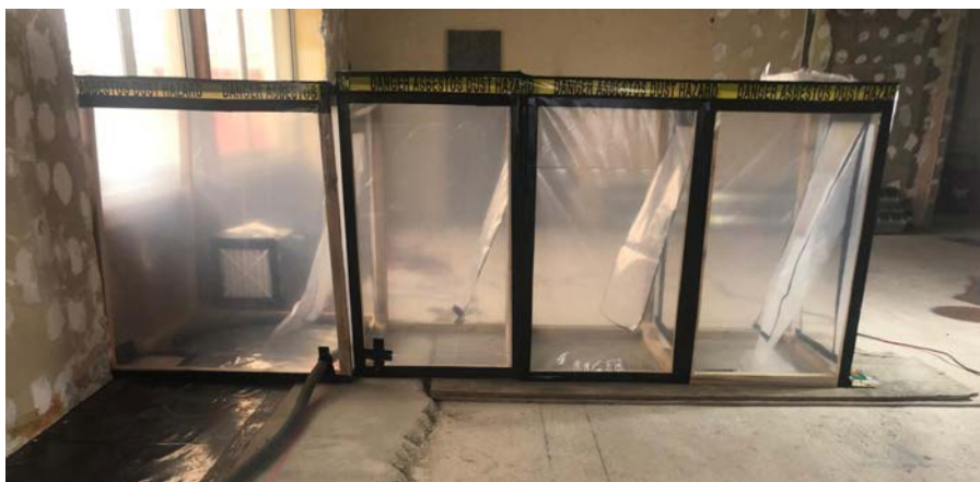
FIGURE 15: Flap arrangements for airlocks
