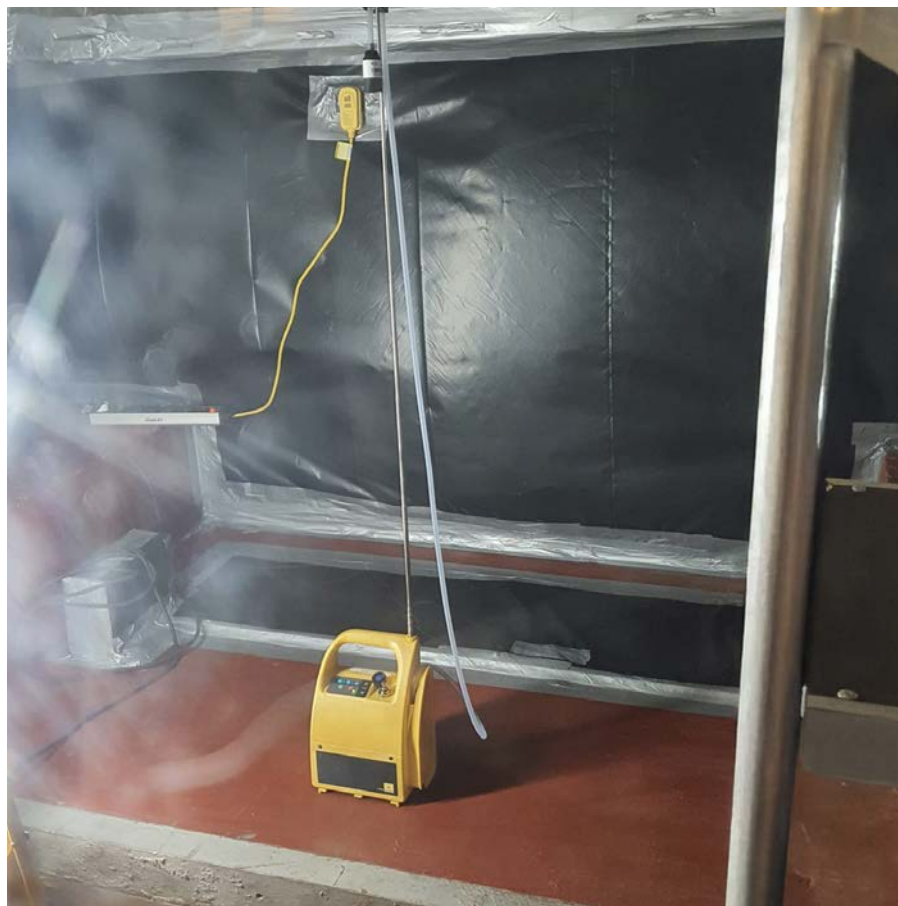
FIGURE 28: Air sampling during clearance (viewed through a vision panel)
