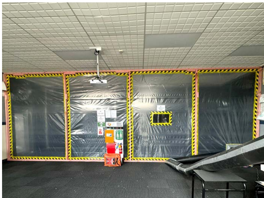
FIGURE 5: Example of a Class A enclosure inside a building
