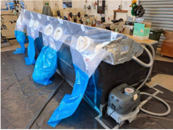
FIGURE 25: Example of glove bag setup with HEPA vacuum
