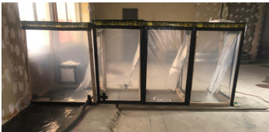
FIGURE 15: Flap arrangements for airlocks
