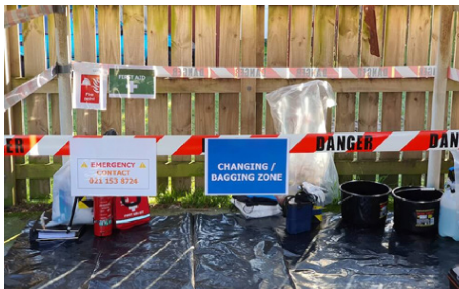
FIGURE 36: Example of preliminary decontamination area when no enclosure present
