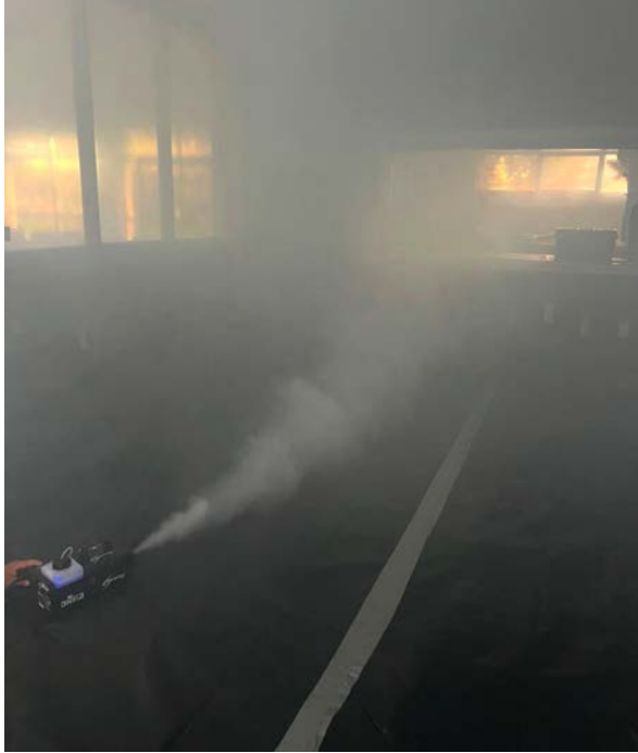
FIGURE 20: An enclosure being smoke tested
