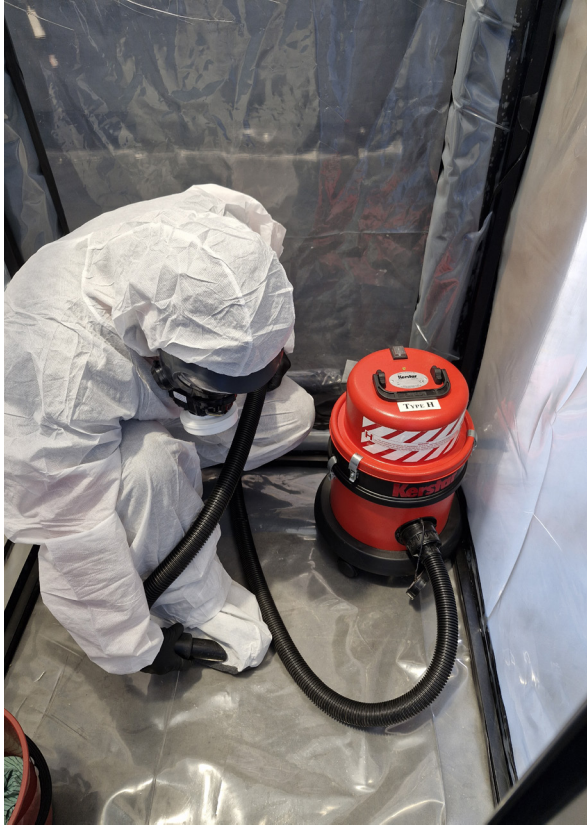
FIGURE 13: Preliminary decontamination with a Class H vacuum cleaner
