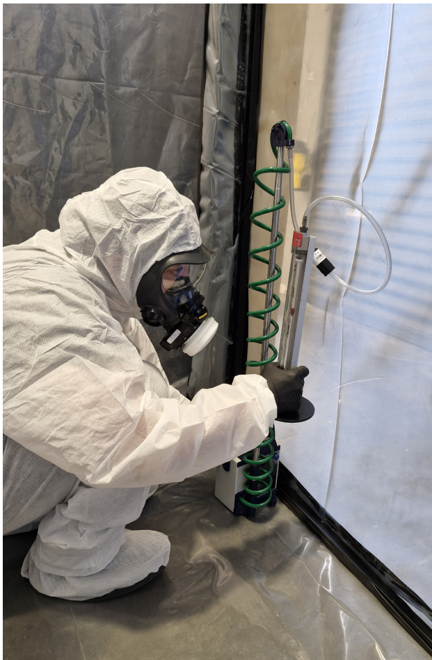
FIGURE 3: Assessor setting up a clearance test
