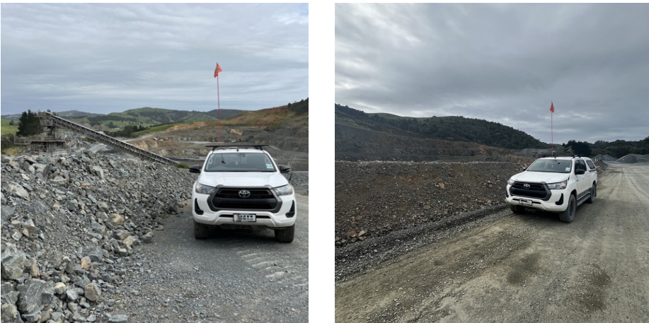
FIGURE 8: Open-edge protection at Whangaripo Quarry (Rodney Aggregates Supplies Ltd)
