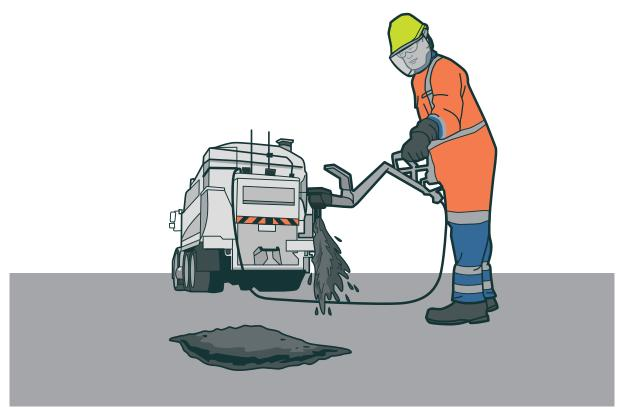
**FIGURE 12:** Example of a worker wearing the correct PPE for the substance being handled
