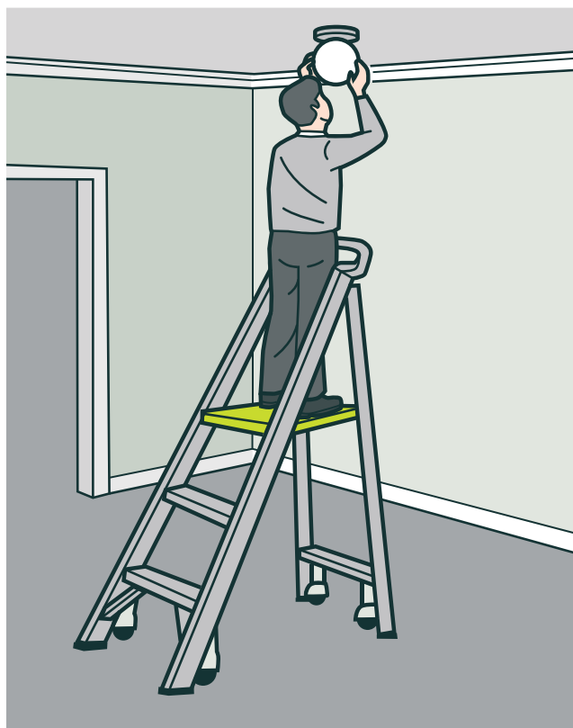
FIGURE 19: A worker uses a step platform
