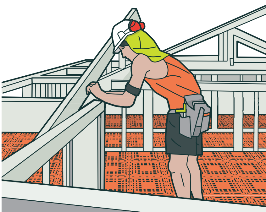
FIGURE 13: A worker standing on a safety deck on a residential building site
