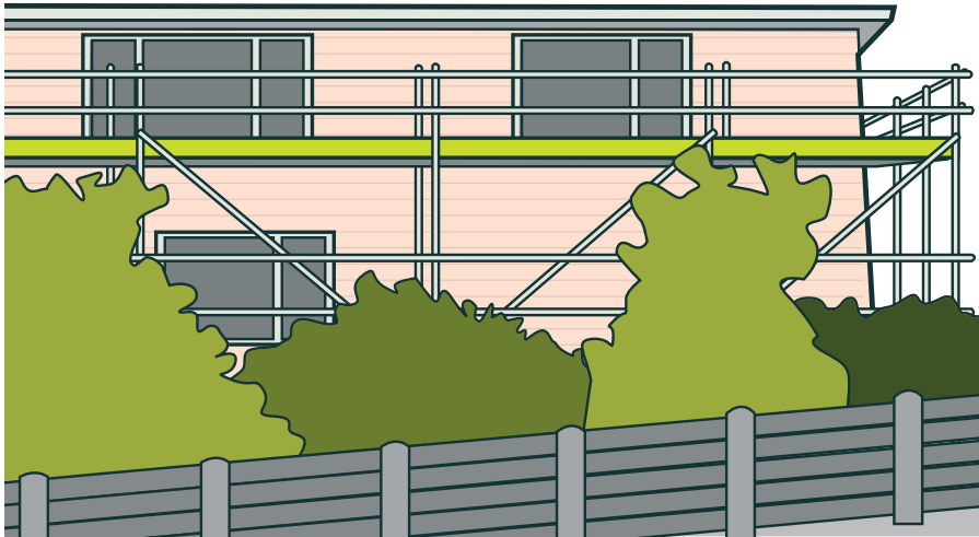
FIGURE 4: Scaffolding on a residential building
