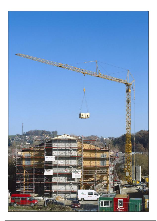
Picture 4: Self-Erecting Tower Crane
