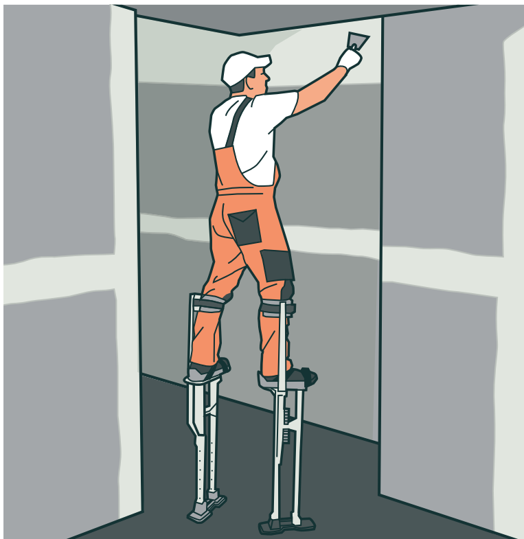
FIGURE 22: A plasterer uses stilts to comfortably reach above doorframes.
