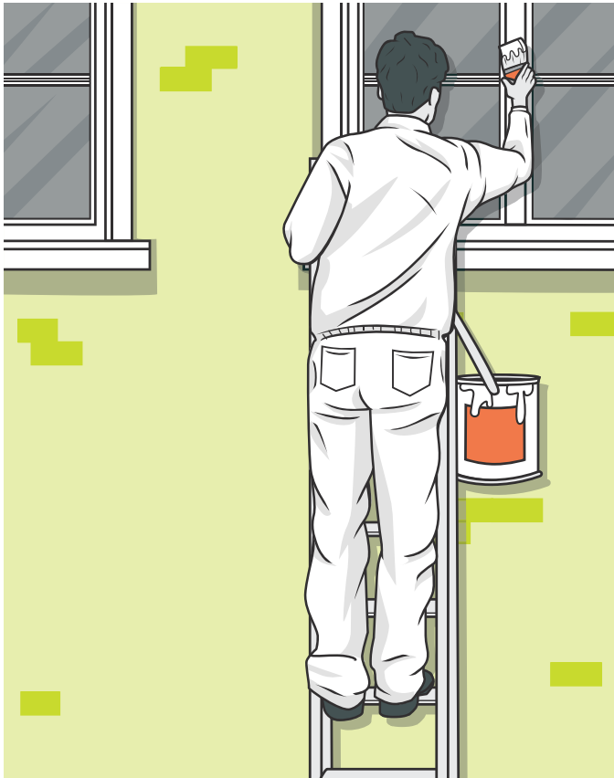
FIGURE 23: Worker maintaining three points of contact with the ladder
