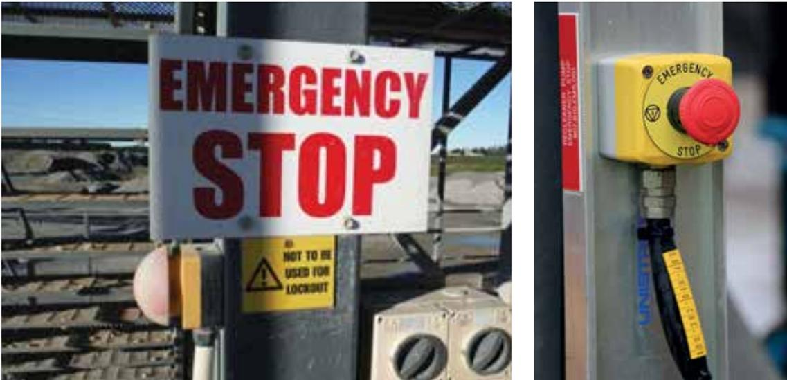
**Figure 88:** Emergency stop with signage (photo courtesy of Fulton Hogan Miner Rd Quarry and NZ Steel Taharoa)
