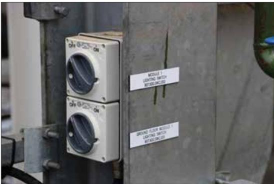
**Figure 110:** Example of an energy-isolating manually operated disconnect switch with a loop for securing a lockout device (photo courtesy of NZ Steel, Taharua)
