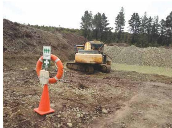
**Figure 102:** Example emergency station Photo supplied by New Zealand Petroleum and Minerals
