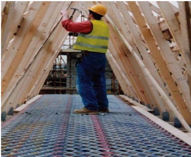
Figure 1: Decking system that provides a working platform in the roof eaves (Image courtesy of Oxford Safety Components Ltd).
