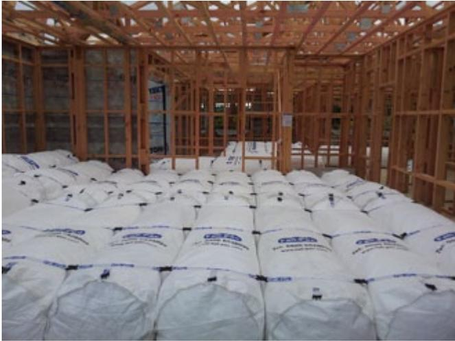
Figure 4: Bean bags being used as a fall mitigation measure during roof work (Image courtesy of Fall-Pac NZ Limited).
