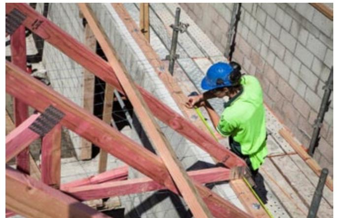
Figure 6: Measuring and installing purlins from an external work platform (Image courtesy of Site Safe New Zealand Inc).
