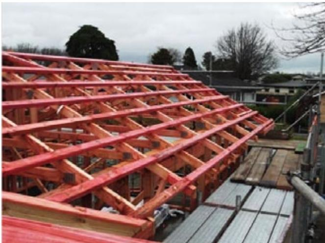
Figure 5: A safe working platform was used at the start of the sequential installation of the purlins/roofing battens.
