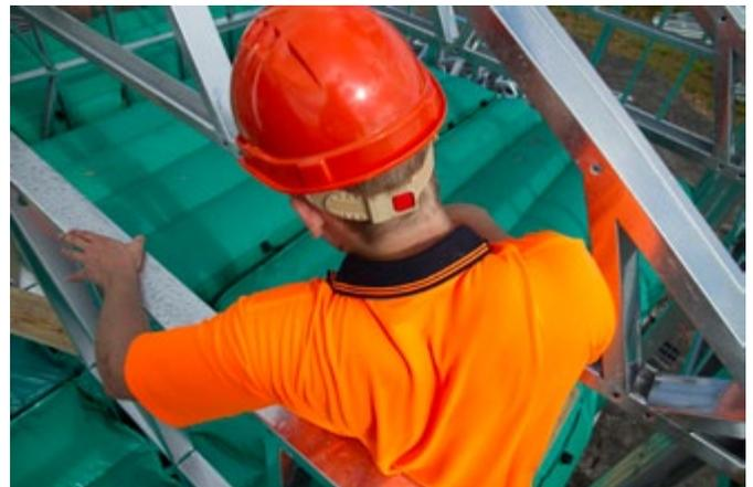
Figure 3: Air bags being used as a fall mitigation measure during roof work (Image courtesy of Airtek Safety Products Ltd).
