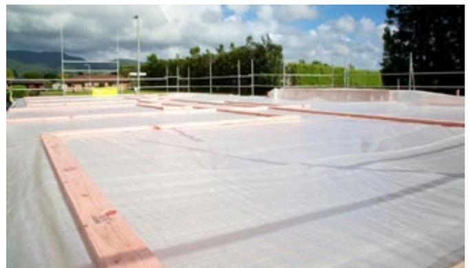
Figure 4: An example of a safety rated product that can span across the top of the framing (image Courtesy of Humpty's Fallbreaker Ltd).
