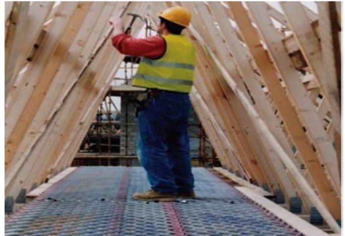
Figure 2: Decking system that provides a working platform in the roof eaves (Image courtesy of Oxford Safety Components Ltd).
