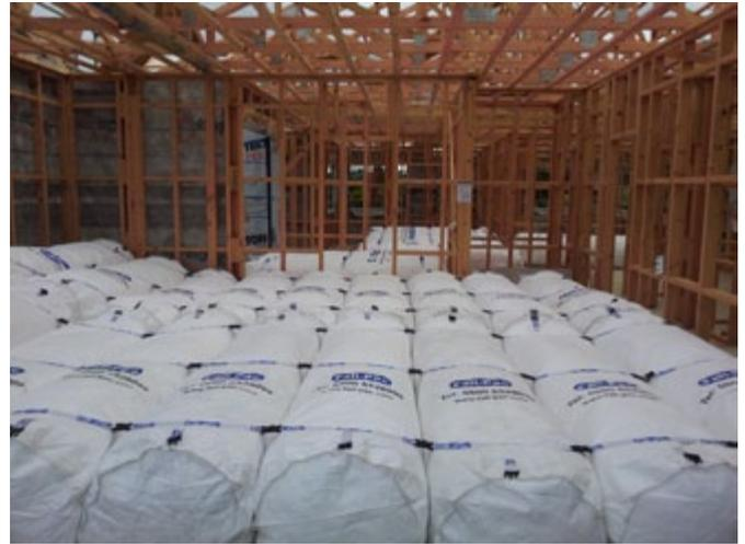
Figure 7: Bean bags being used as a fall mitigation measure during roof work (Image courtesy of Fall-Pac NZ Limited).
