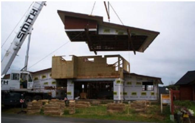
Figure 1: Craning a pre-assembled roof into position greatly reduces the need for work at height (Image courtesy of BJ Carter.)
