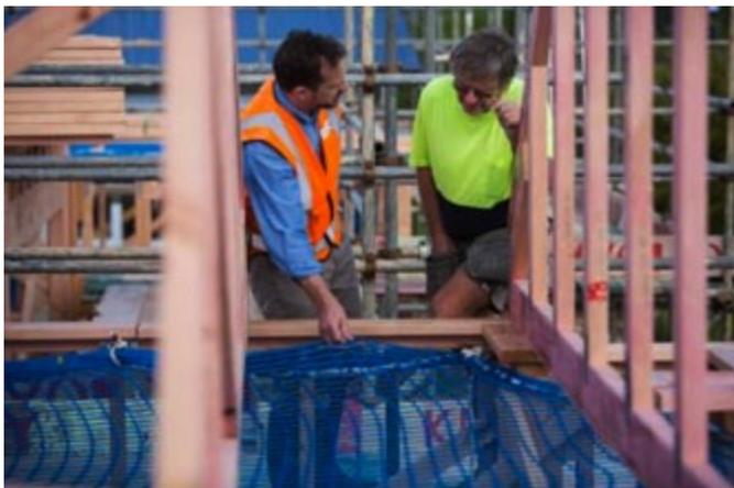
Figure 5: Safety nets installed on a house under construction.
